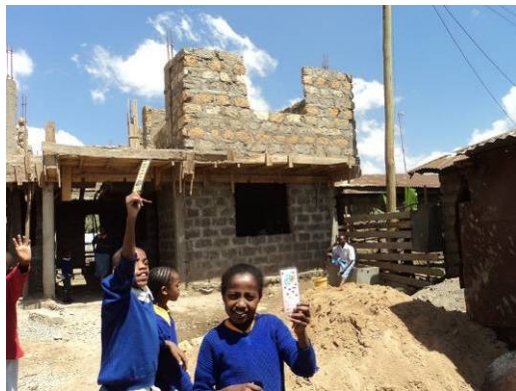
School children in front of the school’s “in progress” construction
